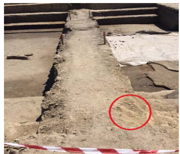
Red circle indicates where the IP lost his footing. Entry ramps were dug by a JCB and then loosely backfilled by hand
