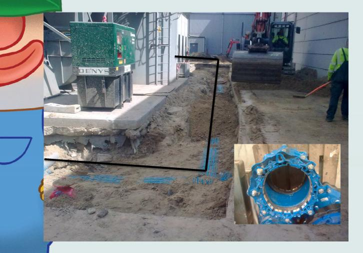
After completing the works, the pipe had to be made operational by the client. During the filling operation (pressure presumably +/- 11 bar) a coupling came loose and moved in the direction of our employees.
