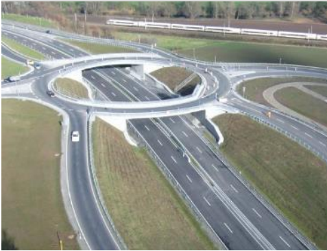
Road Construction and Civil Engineering
