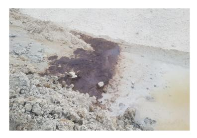
An historical contaminated site have been found along FGP Pipelines 1508/1507/1506 during Trench excavation which was an obstacle to construction works on Pipeline installation. The pollution was very extensive and posed a high risk to the environment and workers' health.
